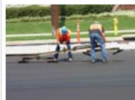
Right of Way Services
